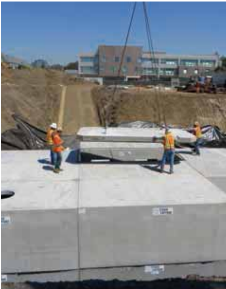
Workers help install StormCapture precast concrete modules. Photo by Oldcastle
